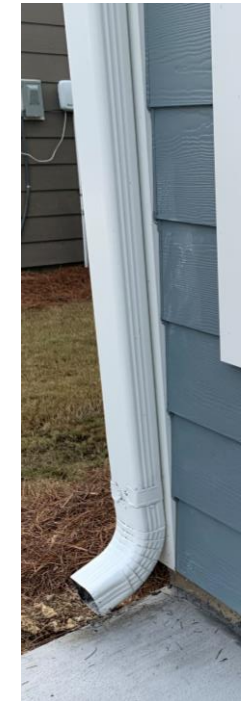
UPGRADES Gutters on front and rear of house.
