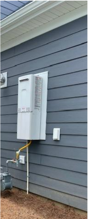
EXTERIOR TANKLESS WATER HEATER
